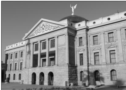
Many state legislatures have outgrown their historic buildings, such as this state capitol building in Arizona.
